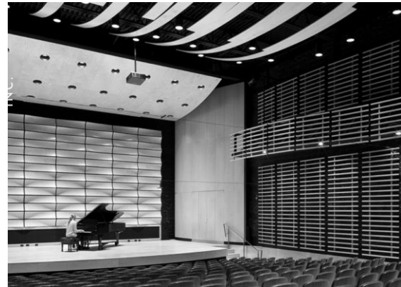
Figure 3: von Kuster Hall, University of Western Ontario. What looks like a side wall balcony is an unoccupied "shelf" used to generate beneficial lateral soffit reflections.
